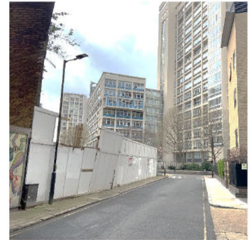
Looking southwest from under the viaduct on Tiverton Street
